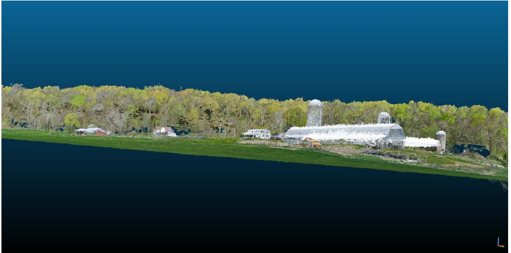
Figure 10. Photogrammetrically derived “point cloud” generated from imagery taken by UVM SAL’s unmanned aircraft system, facing west from landward approach.
